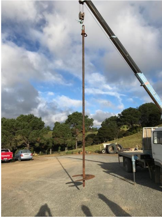
Figure 5a: Screw anchor overview
