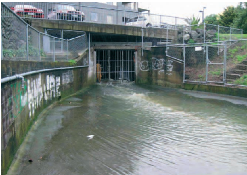
Figure 15: Combined wastewater and stormwater overflowing from a constructed discharge point following a heavy rainfall event.
