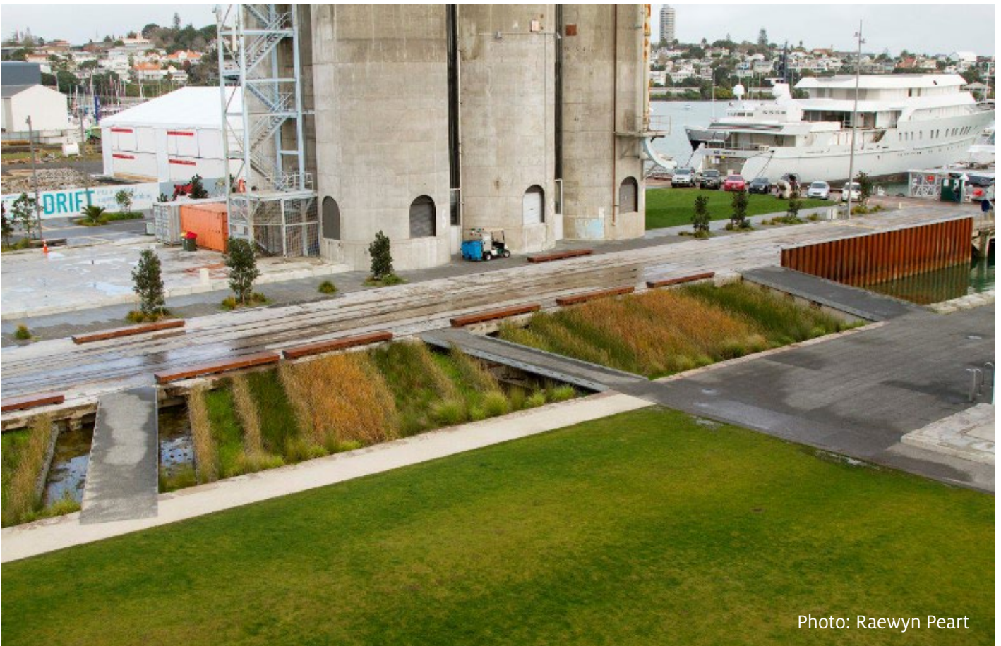
Figure 7.5 Green infrastructure – Constructed wetlands at Wynyard Quarter
