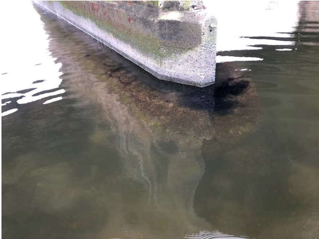
Figure 4.2. Australian tubeworms ( Ficopomatus enigmaticus ) are present from the low water mark to near the riverbed on every pile of the bridge that is in the water.
