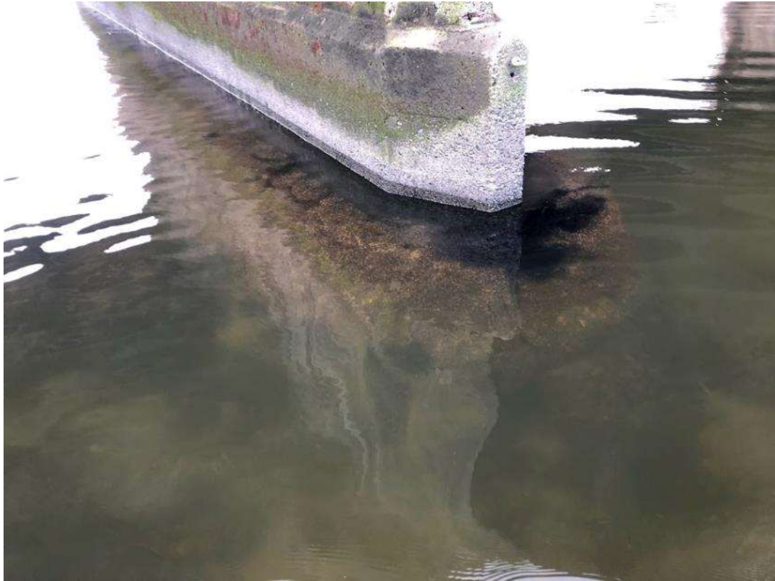
Figure 6-13. Australian tubeworms ( Ficopomatus enigmaticus ) are present from the low water mark to near the riverbed on every pile of the bridge that is in the water.
